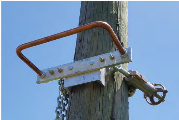
Cluster Bar without penetrating feature
