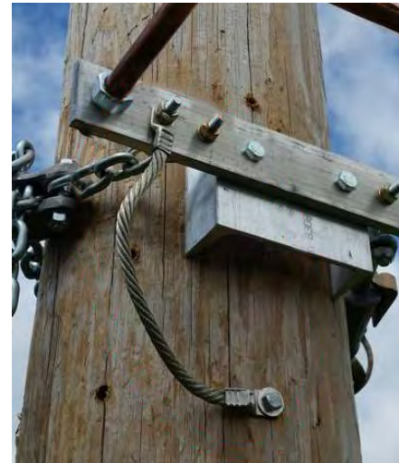
Cluster Bar with penetrating feature
